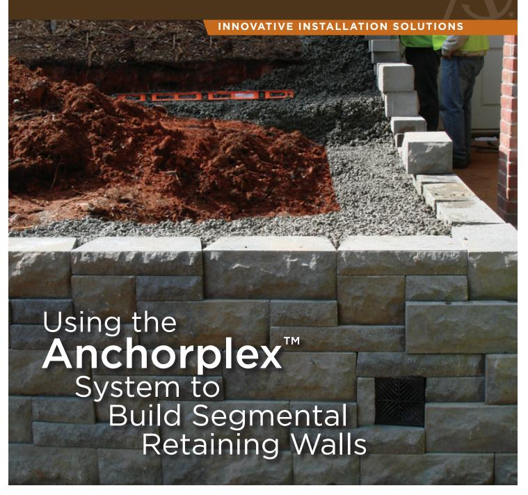
The Anchorplex™ retaining wall system offers a unique, nonconventional solution to difficult-site wall construction problems. The Anchorplex system is a retaining wall built with Anchor™ products and self-compacting structural backfill specified by Anchor Wall Systems, and backed by engineering support tools developed by Anchor Wall Systems.
